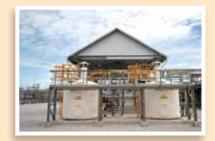
Odor Treatment Plant (OTP), involving OTP blowers and activated carbon filter units, is installed to minimize odor in WWTP. All odor concern process areas, including Equalization tank, Diversion tank and Bio-reactor basins, are covered. The air from these process are used as alternative air in the biological treatment. The excess air will be treated by activated carbon filter unit. Since the first start up of OTP, there has never been any odor issue in WWTP.
